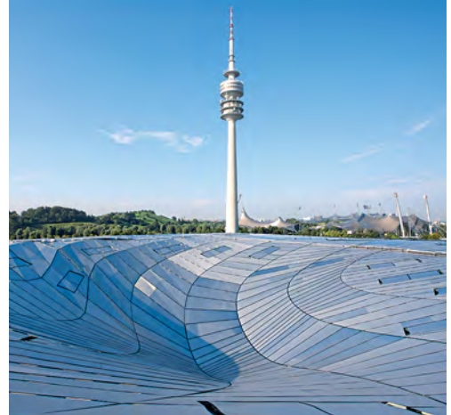
Even the roof of the double cone, curving in- wards in the shape of a tornado, is also covered with stainless steel sheet.
