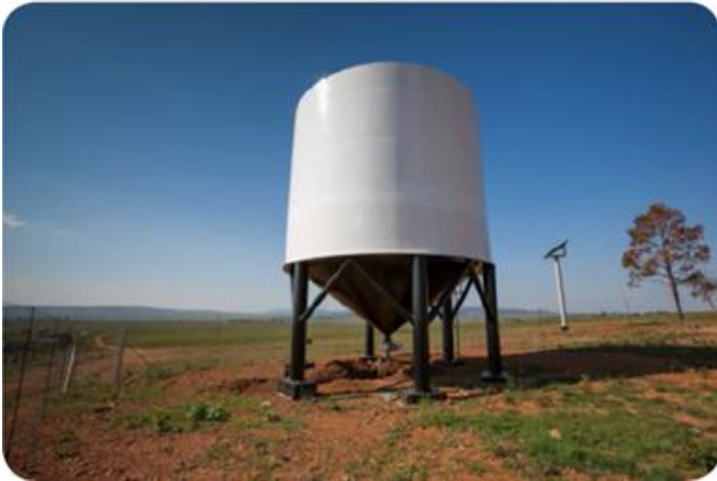
Municipal water tank manufactured from 3CR12 instead of concrete; the manufacturer won an award from SASSDA
